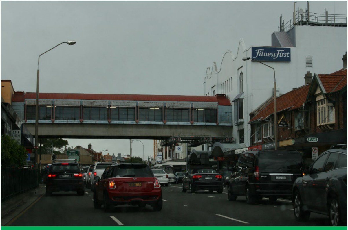
Original Bridgepoint Pedestrian Bridge
