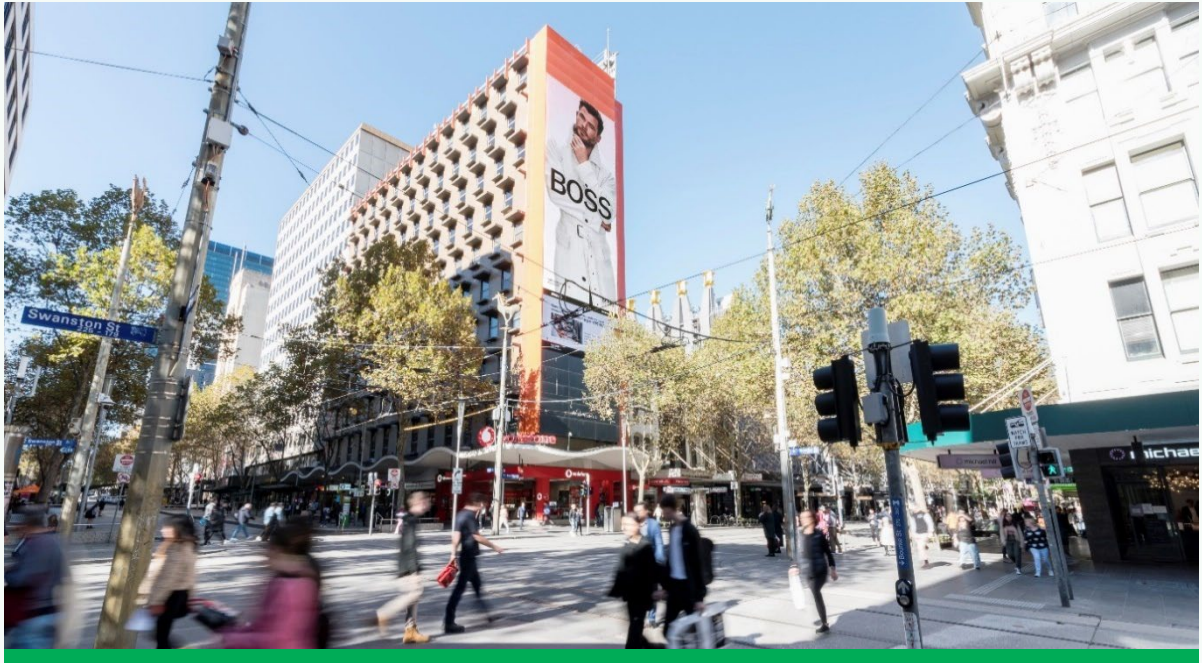
Bourke Street New Digital Display
